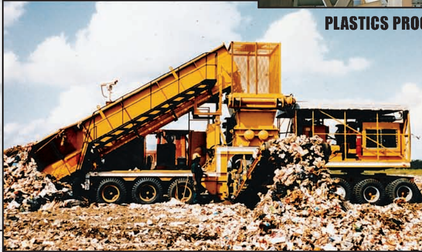
MSW SHREDDING (ONSITE)
